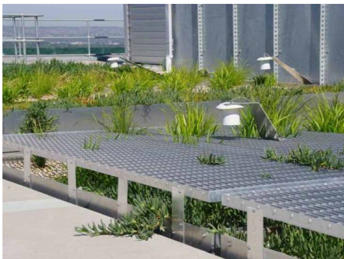
Figure 6. Experimental green roof systems on the roof of ANZ House, Adelaide.
