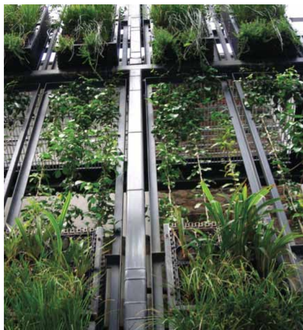
Figure 7. A hybrid living wall in Adelaide incorporates green wall modules and green facades grown in containers.
